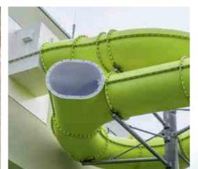
Fake Slide elements provide the guest with an optical illusion that feigns the straight run of the slide, although the actual alignment runs as a curve.
