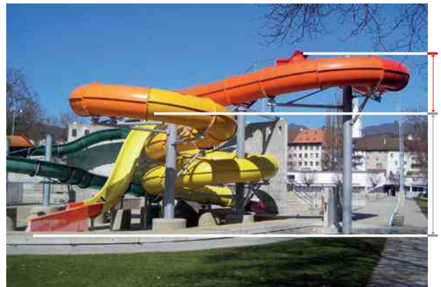
Example of the modernization of a water slide park in Olten, Switzerland. Existing foundations and steel supports were re-used for the new tracks. The previous 40m open slide was transformed into a 75m enclosed tube slide; a new attraction with an excellent cost-value ratio.
